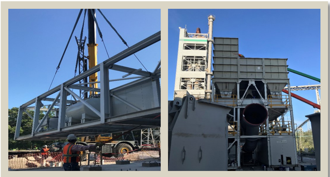
Figure 3: Containerized modules with integrated steel construction
