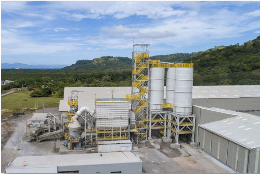
Figure 2: ready2grind plant R2G equipped with an MVR mill 2500 C-4 in Caldera, Costa Rica
