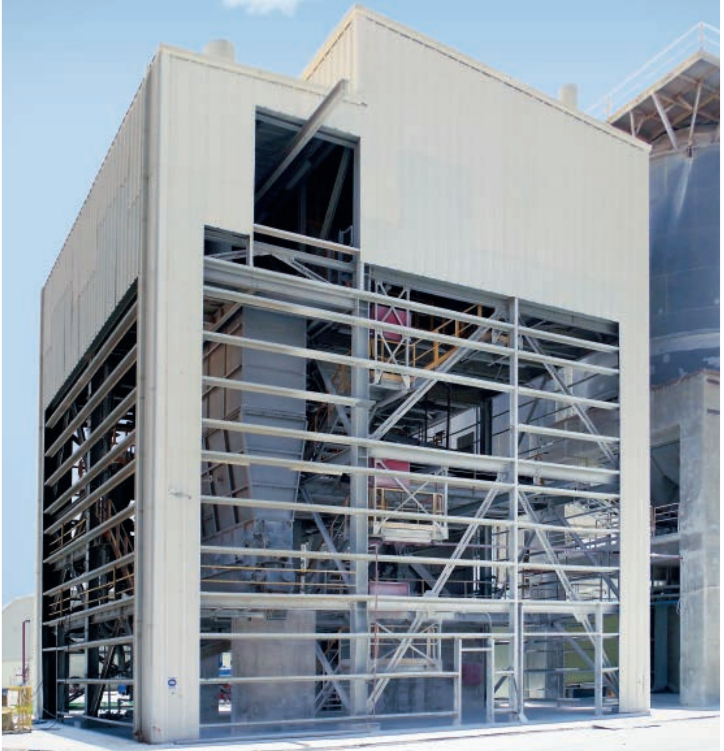
Lime hydrating plant in Saudi Arabia including SLV high-efficiency separator , MRD ball mill and KLV lime hydrator
